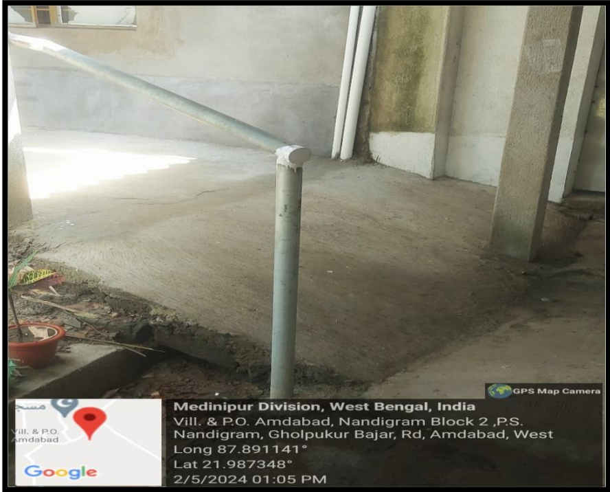
Slope/Ramp has been made in Different Step down Parts of the Campus along with Railings
