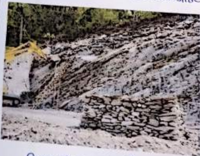
Rock Slope Netting
