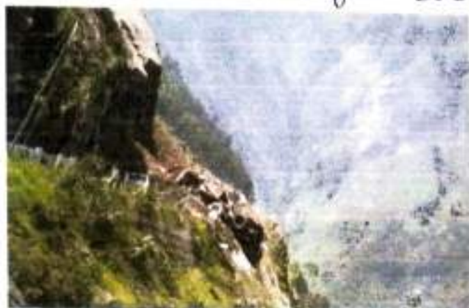
7. Namchi-Pabongla road was closed due to landslide
