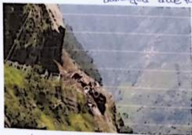
Namchi - Rabongla road was closed due to landslide
