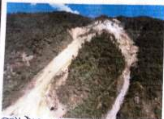
Peshing village in Namchi district due to landslide
