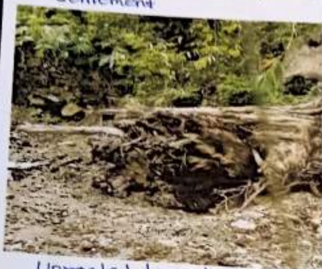
Uprooted tree due landslide
