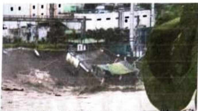
The IPCA laboratory was badly affected due to landslide
