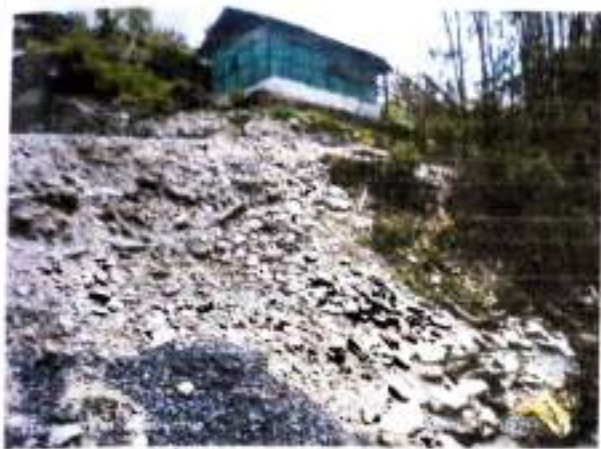
1. Landslide prone area, unplanned settlement.
