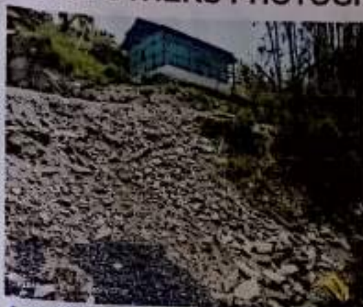
Landslide prone area, un-planned settlement
