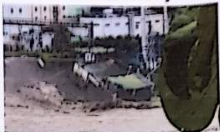
The IPCC laboratory was badly affected due to landslide
