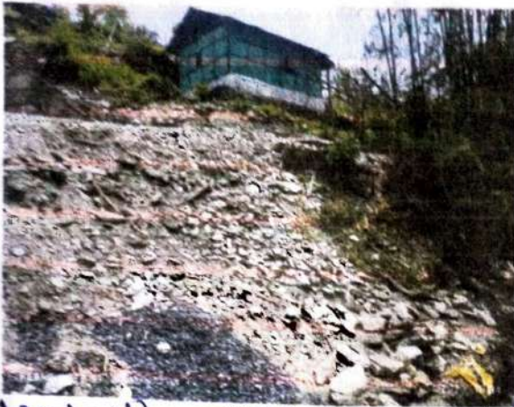
landslide prone area on plain near settlement
