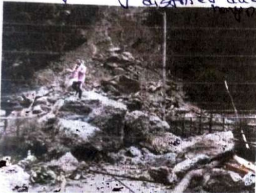
Tista stage dam was broken due to landslide
