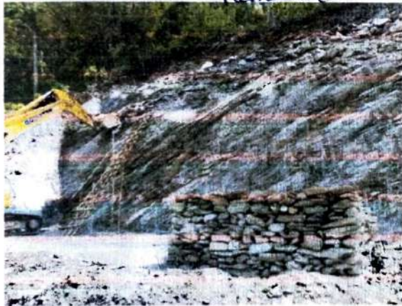
Rock slope netting
