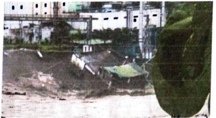
The IPEA laboratory was badly affected due to landslide
