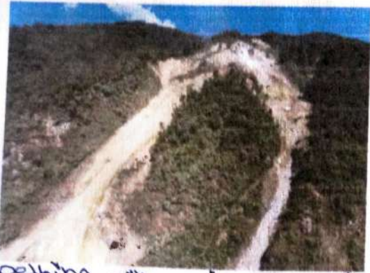
Pething village in Namchi destroyed due to landslide
