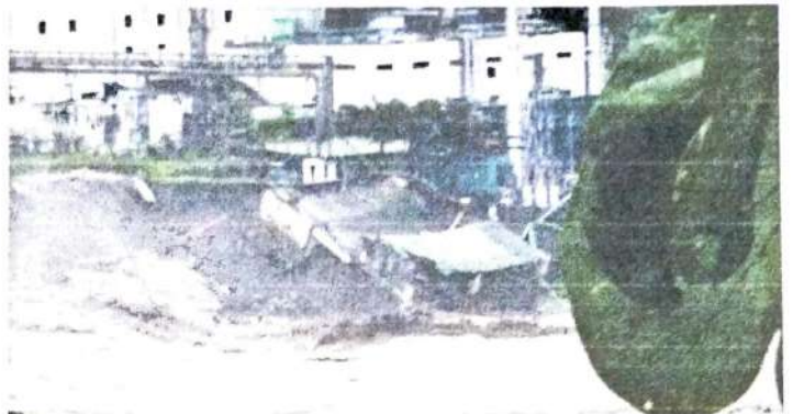
The IPCA laboratory was badly affected due to landslide
