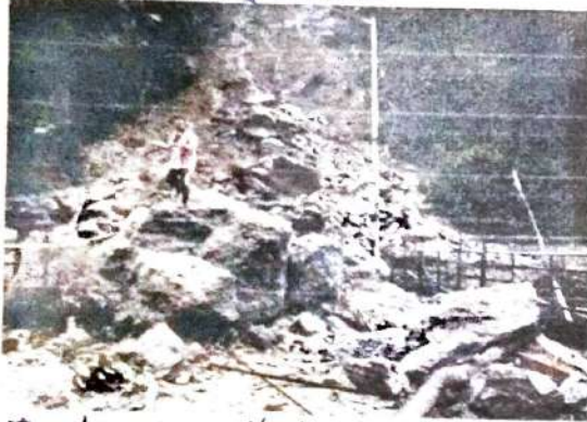
Teesta stage-V dam was broken due to landslide
