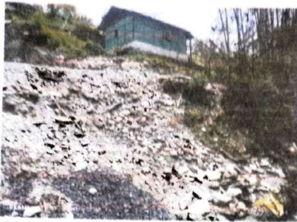
Landslide prone area unplanned Settlement
