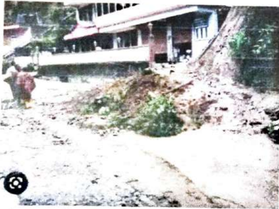
14 people died in pelling due to landslide
