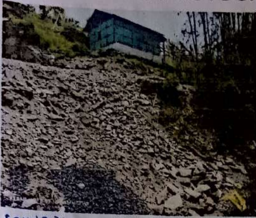
Landslide prone area, un-planned settlement
