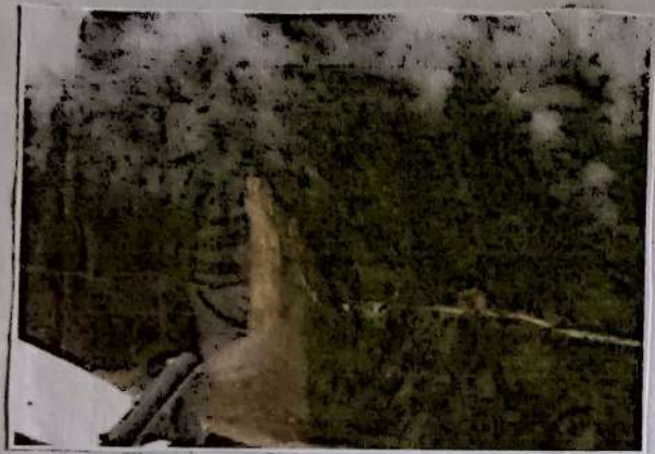
Landslides all over Sikkim due to earthquake
