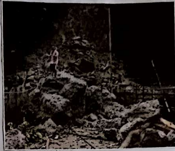
Teesta Stage-V dam was broken due to landslide
