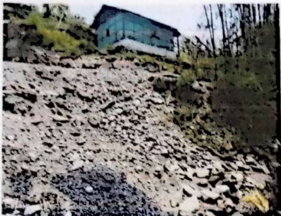
Land slide prone area unplanned settlement
