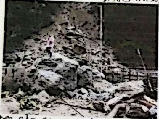
The stone stage - dam was broken due to landslide.
