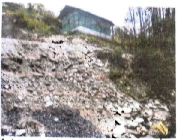
1. Landslide prone area unplanned settlement
