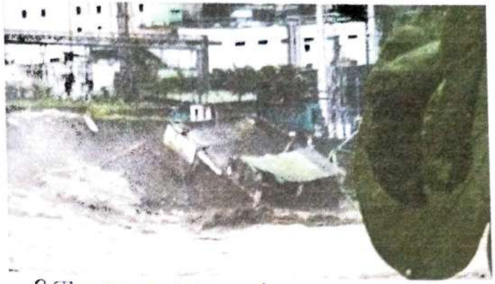
2. The IPCC laboratory was badly affected due to landslide
