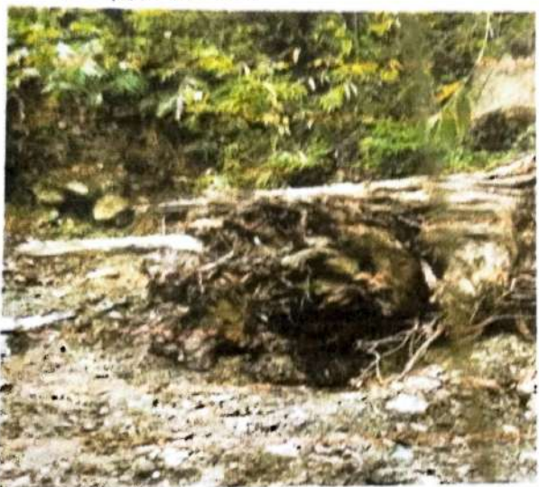
3. Uprooted tree due to landslide
