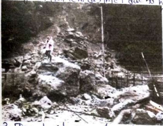
3. Teesta stage - v dam was broken due to landslide
