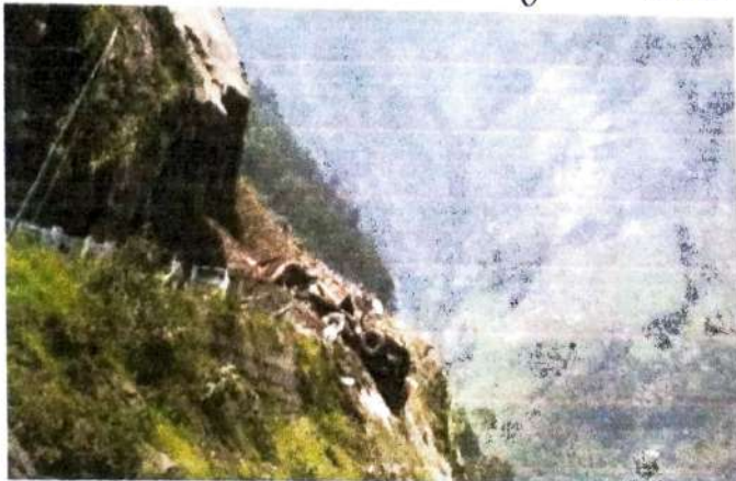
7. Namchi - Rabongla road was closed due to landslide
