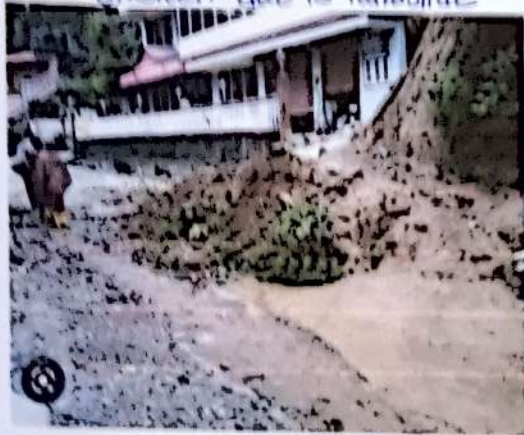
14 people died in pelling due to landslide
