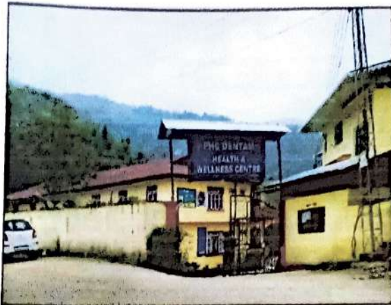
Primary Health center in Dentham valley
