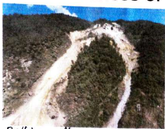
Pathing village in Namchi district due to heavy rainfall
