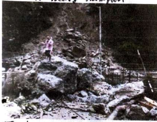
Testa Stager-v dam was broken due to landslide
