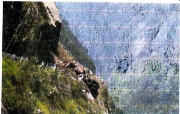
Namchi - Rabangla road ways closed due to landslide
