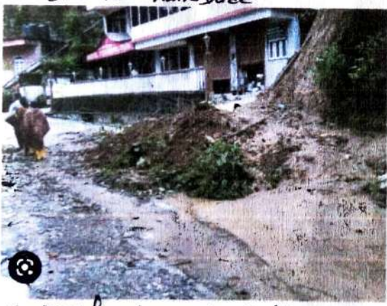
14 people died in pelling due to landslide
