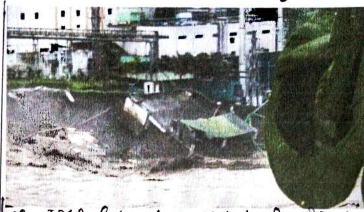
The IPCA laboratory was badly effected due to landslide
