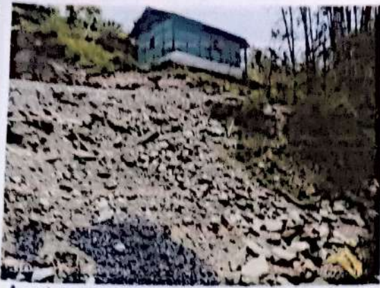
landslide prone area unplanned settlement
