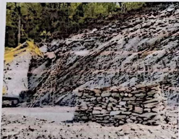
Rock Slope Netting
