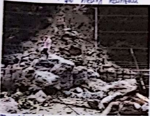
Teesta stage-r dam was broken due to landslide
