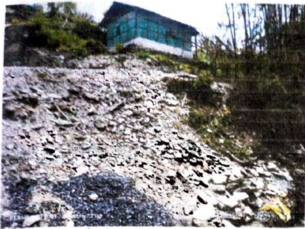
1. Landslide prone area. unplanned settlement.
