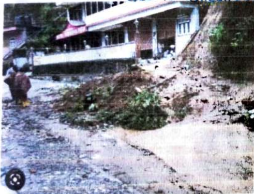
5. 14 people died in pelling due to landslide.
