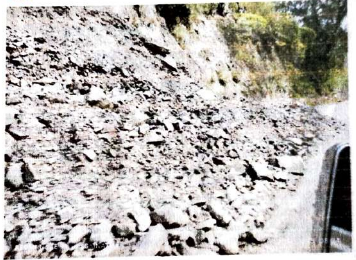
4. Subsidence of slope.
