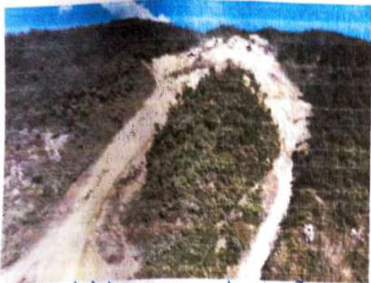
1. A landslide occurred at Pathing village in Namchi district due to heavy rainfall
