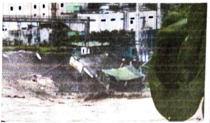
2. The IPCA laboratory was badly affected due to landslide
