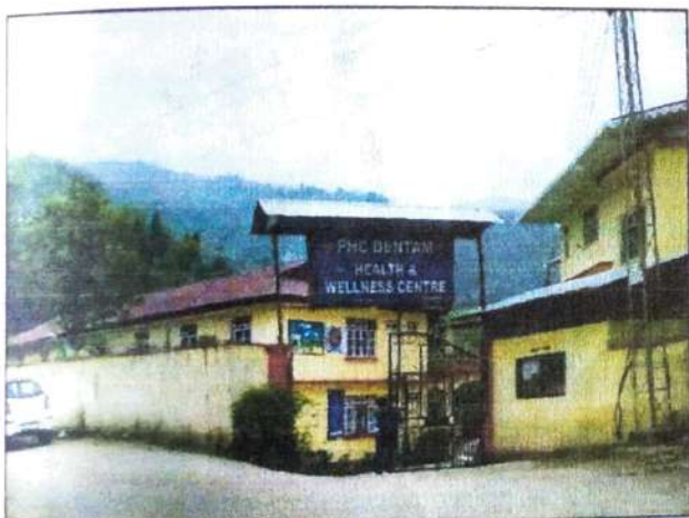
3. Primary health center in DENTUTT
